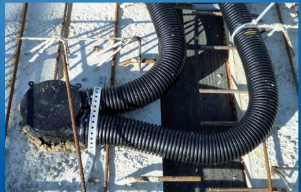
The installation in the unfinished concrete ceiling requires only few elements; the tight bending radius of the pipes allows for an installation without additional shaped parts.
